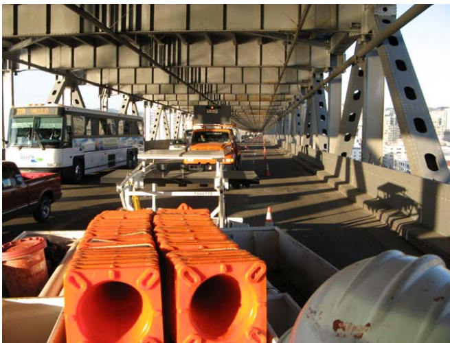
Figure 1 – Caltrans lane closure on Bay Bridge April 2007
